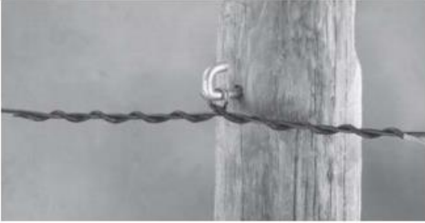
Figure 2: ADSS Tangent Drop Cable Support
